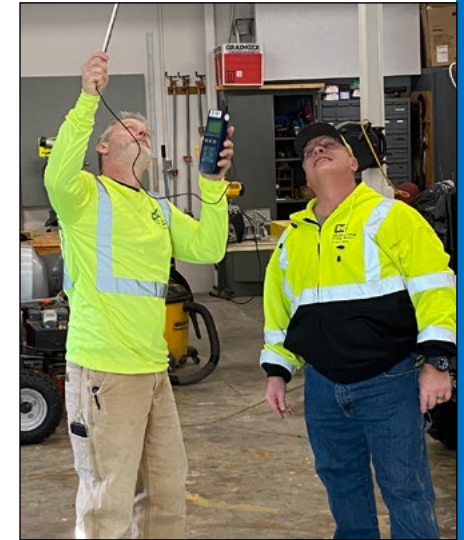
(left) Dustin Strand, safety and occupational health specialist, and John Dehnke, collateral duty safety officer, sample the ventilation system at Lock and Dam 5 near Minnesota City, Minnesota. USACE St. Paul District courtesy photo
